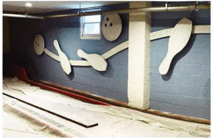
The lanes as they underwent renovation
