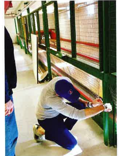
Let the renovation begin!
